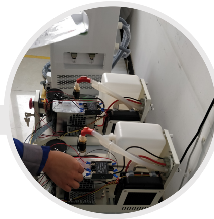
Second inspection Electrical line inspection
